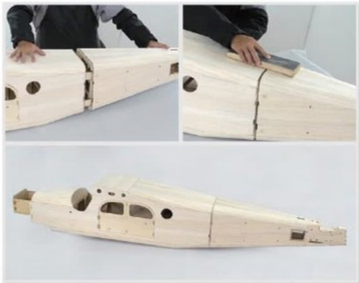
4.34 Trial fit tail section to front section and sand down joining area.
